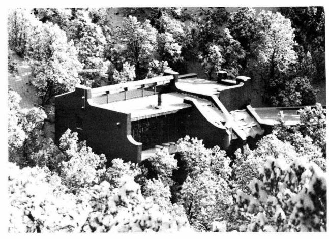
BOB HARNAR (7417) took this picture of his passive solar adobe house in the Sandias after a snowfall last winter. A large clerestory and solar greenhouse are features of the south-facing facade. Note horseshoe-shaped entryway, which holds a solar collector for the hot water system on the roof. Garage workshop extends to the right behind the trees.
